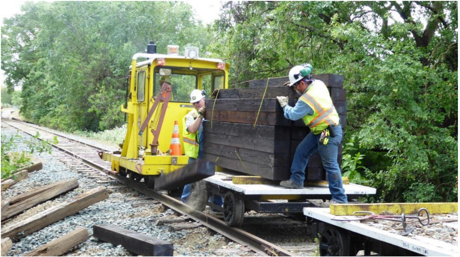
Chris and Joe deploy new ties
