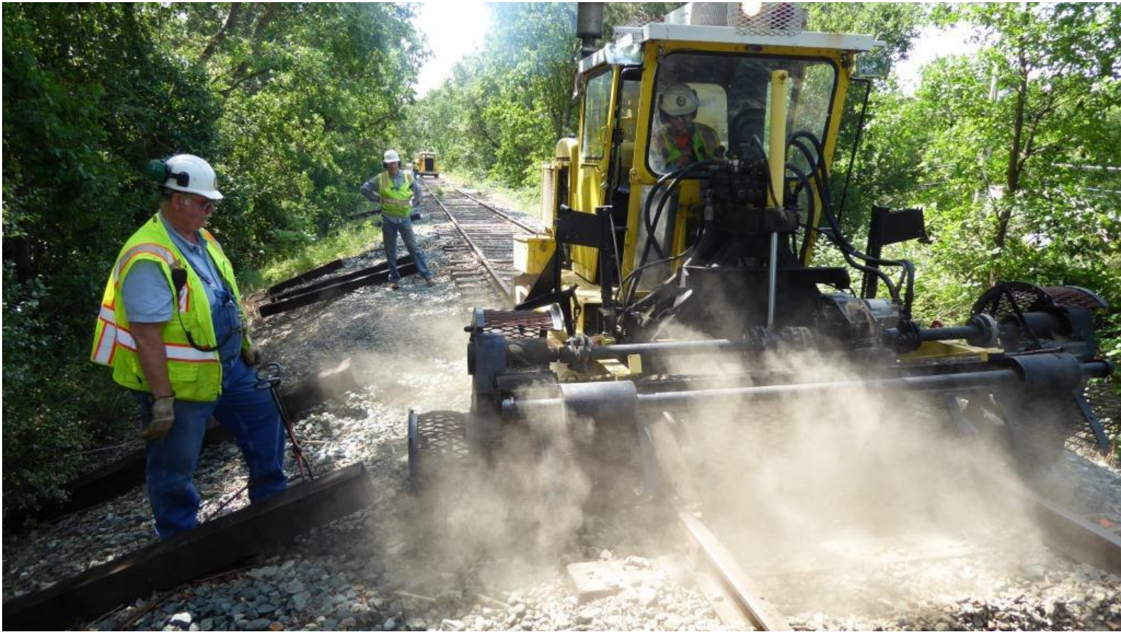
Chris stand ready with a new tie as Joe in the scarifier digs a fresh tie-crib
