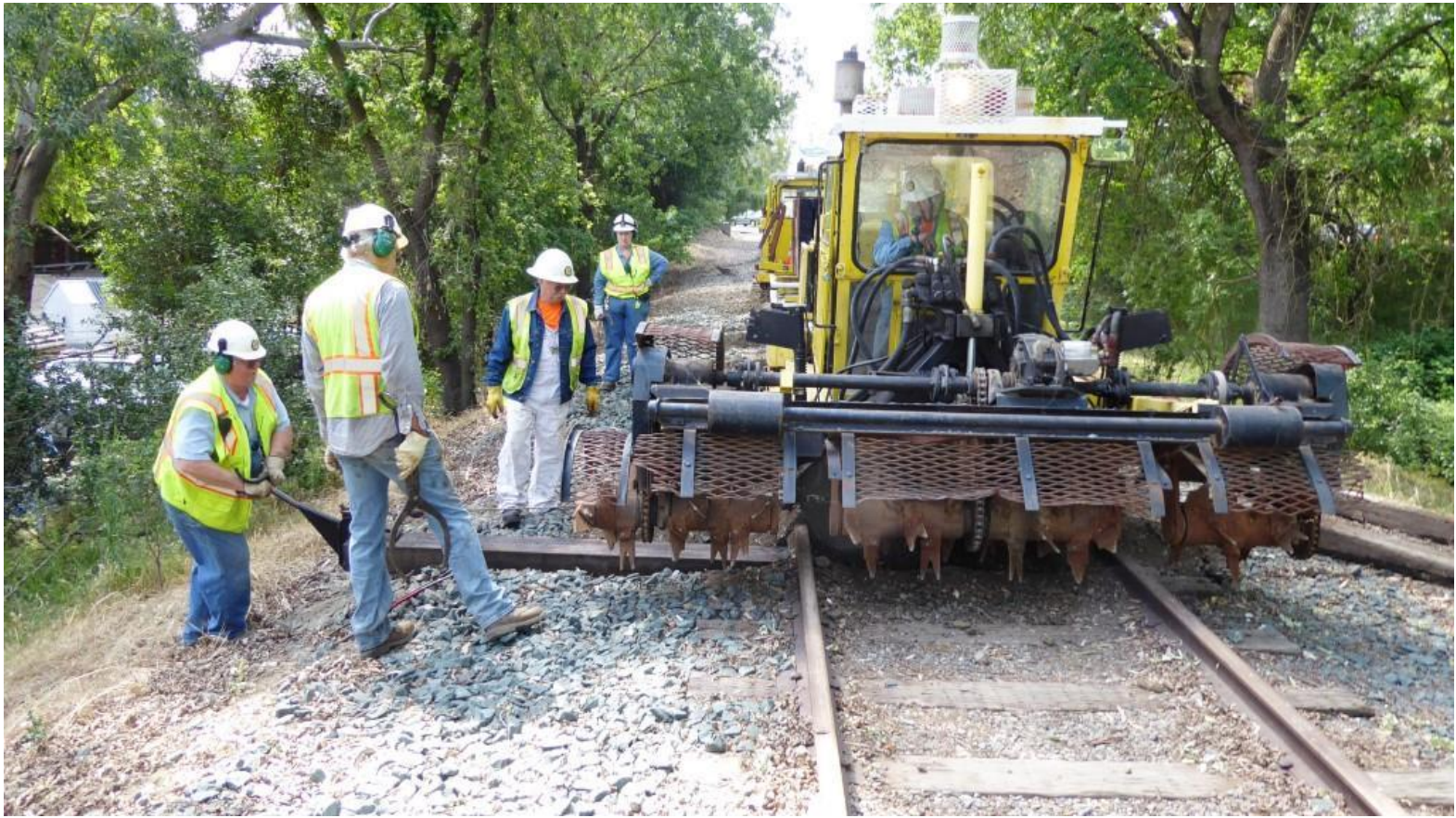
Chris guides a tie into place as Joe pulls it in with the scarifier-inserter's wench
