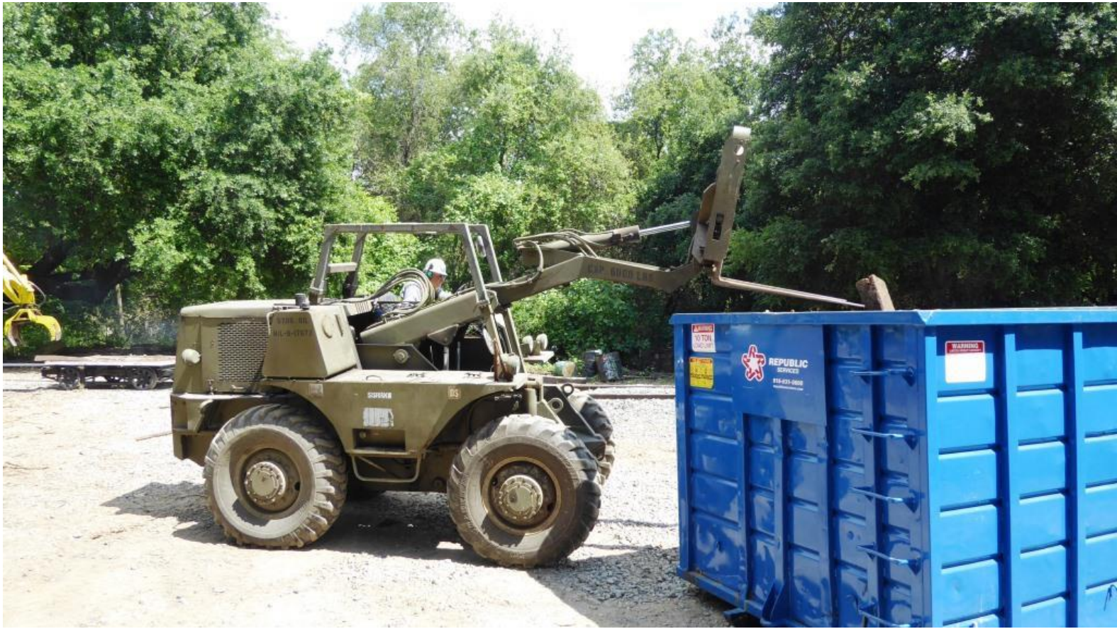
Steve skillfully uses GM2's forks to push a wayward tie into place
