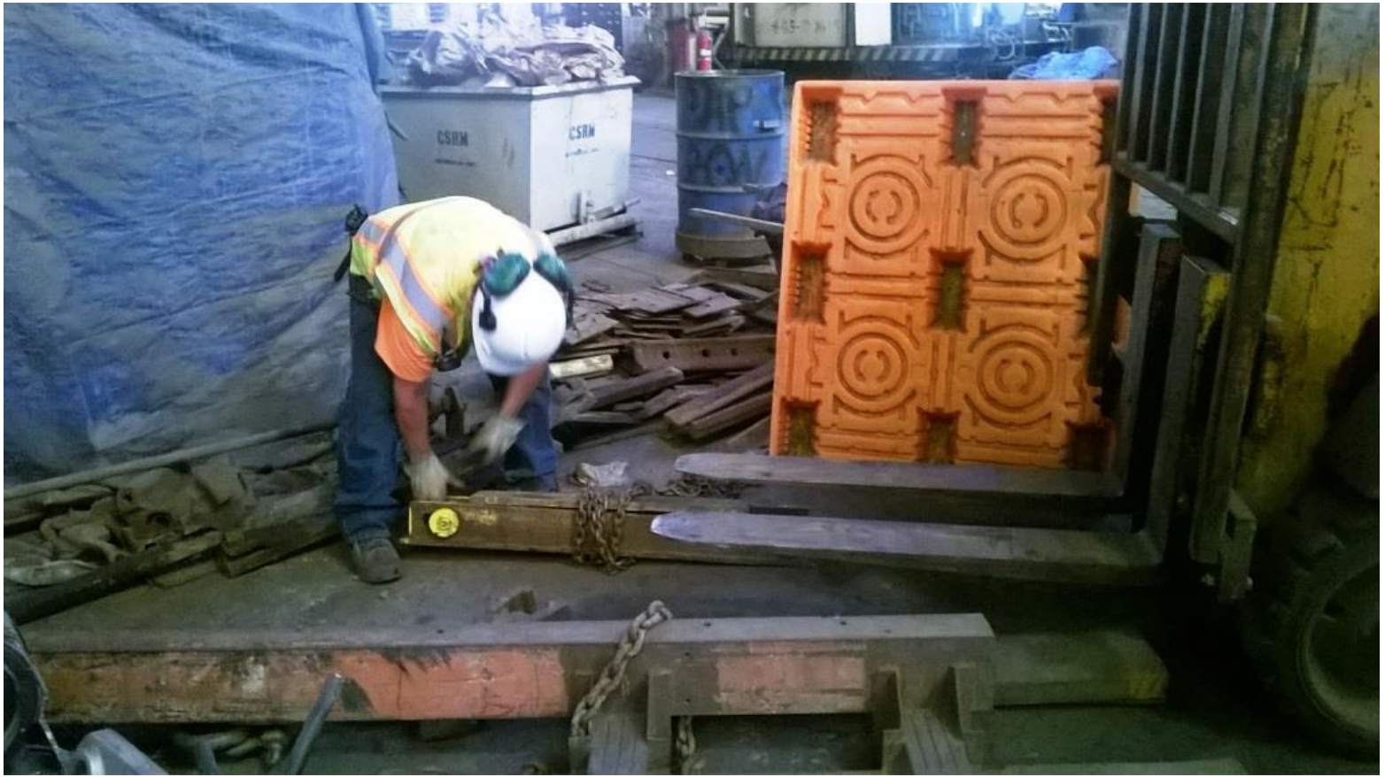
Joe assesses the damage to the lifting ram from the Jackson 125
