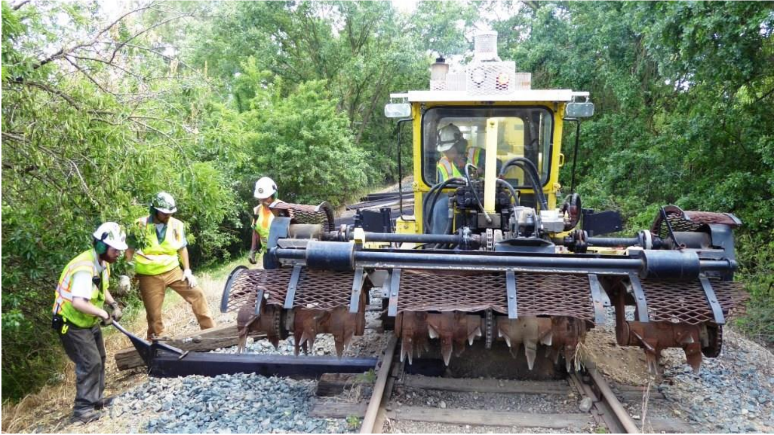
Matt guide a new tie as it is pulled into place under the rails
