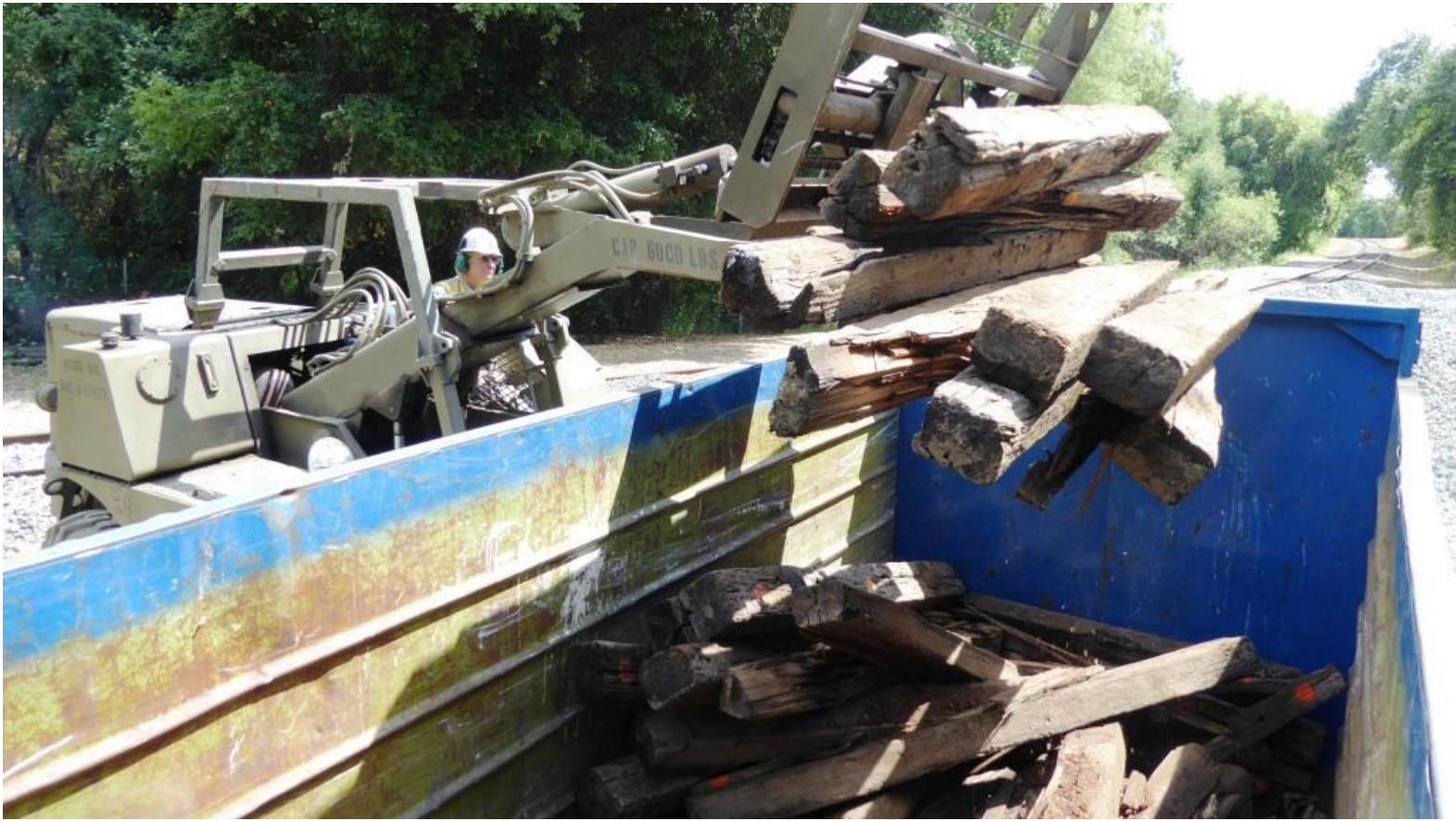
Steve on GM2 drops more dead-ties into the dumpster
