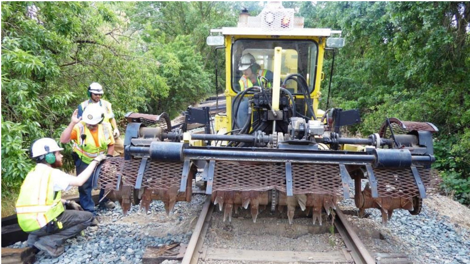
Joe guides Heather in the scarifier to the right spot for pulling in another tie
