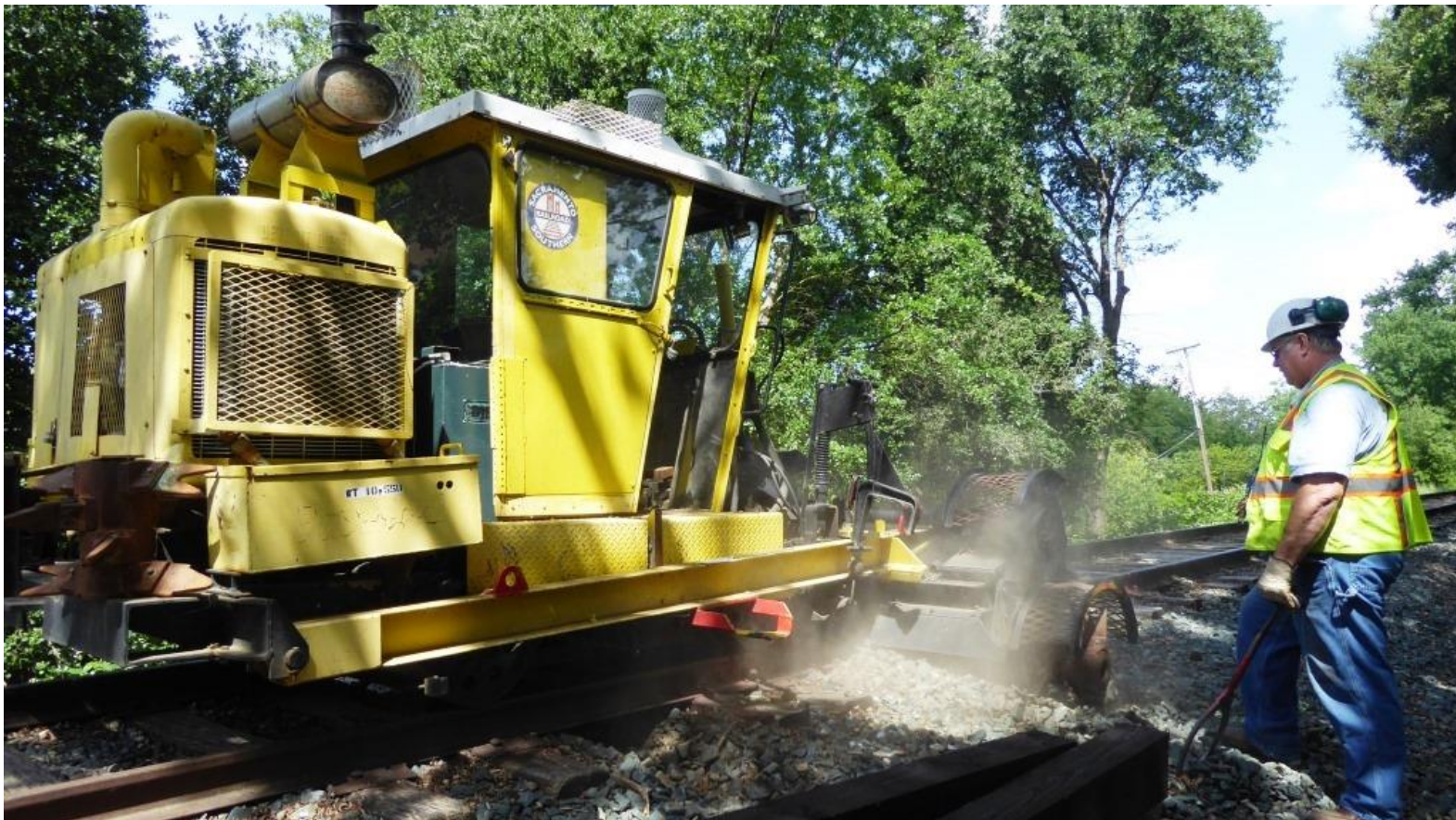
The scarifier scarifies the tie-crib
