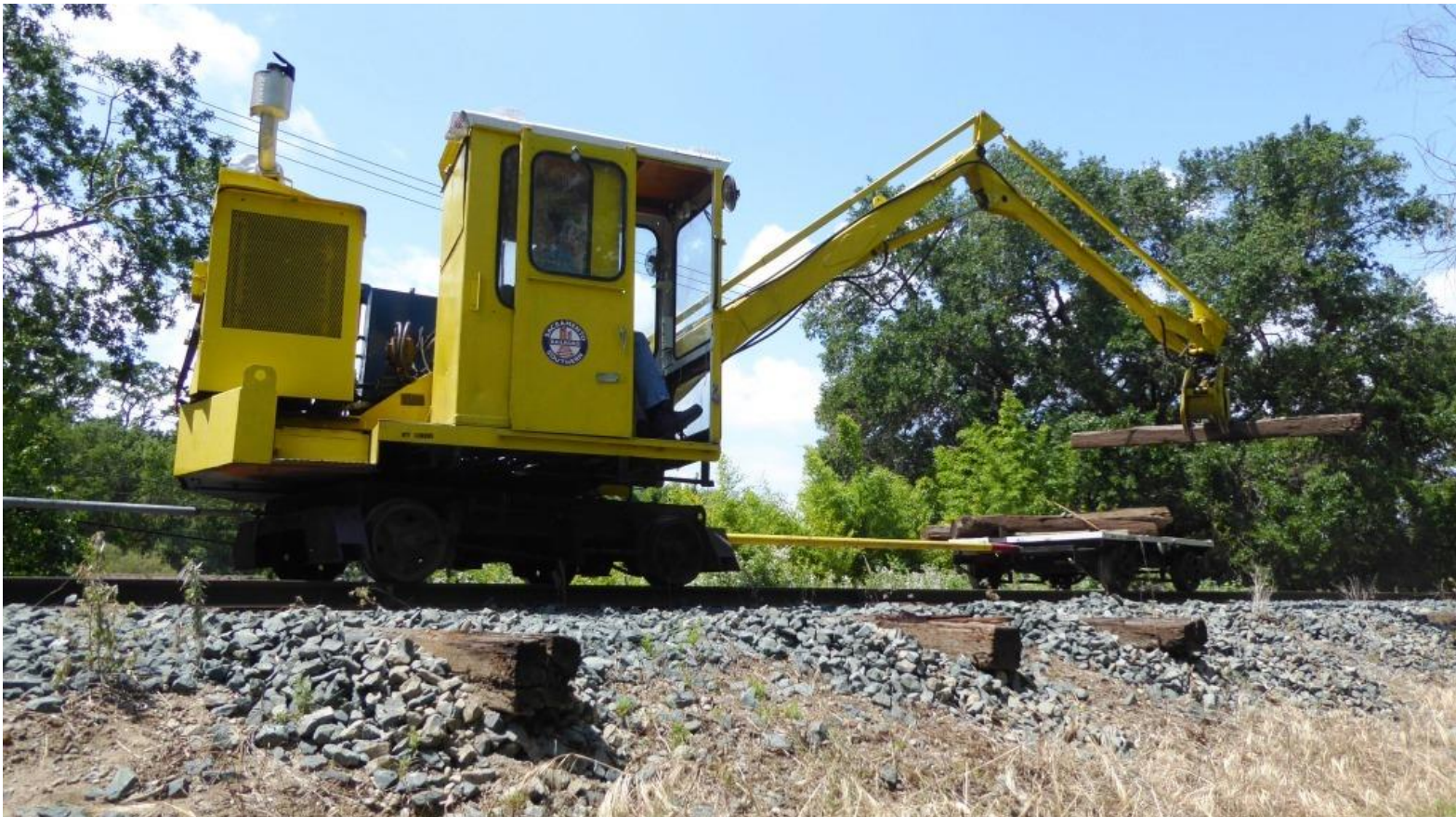
Alan grabs dead-ties with the tie-crane
