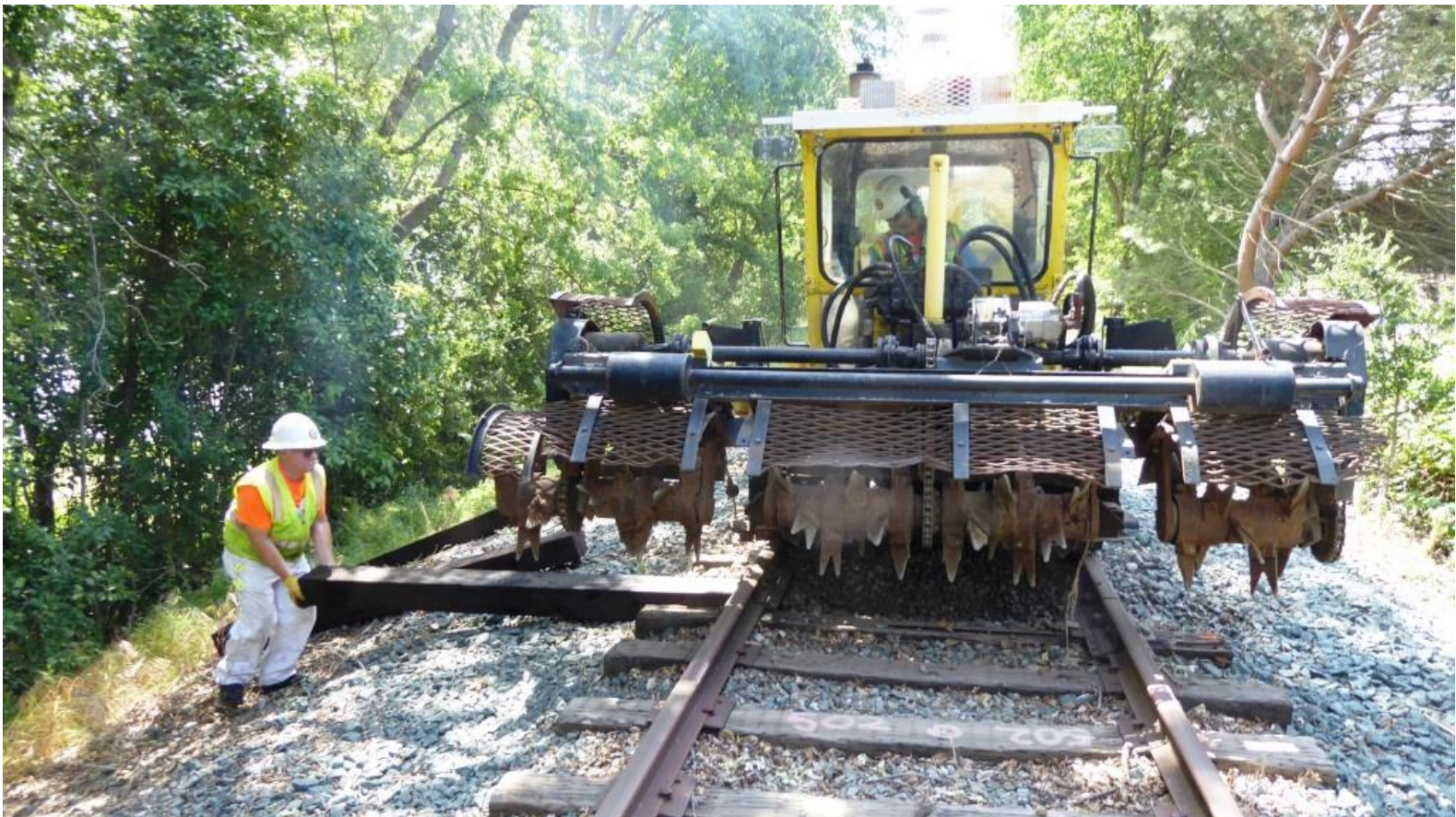
Mike H. positions a tie to be inserted
